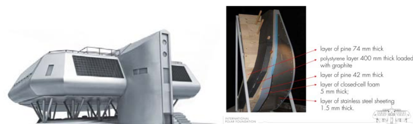
Fig. 8 - the Princess Elisabeth Antarctica and its exterior wall Assembly
